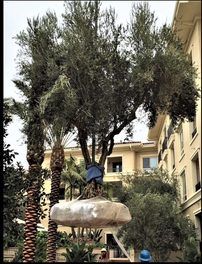
Basket rig using crane
